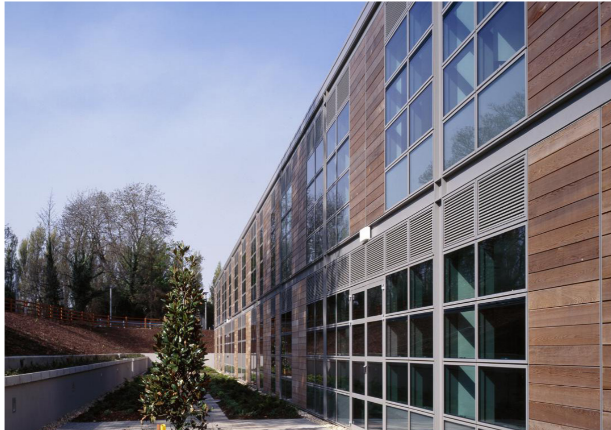
Reference : Exposed Metal Detailing, St Vincents Hospital, STW Architects
